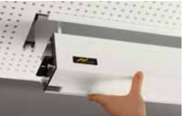
Service-assembly of roll-up screen at the end of building works.
